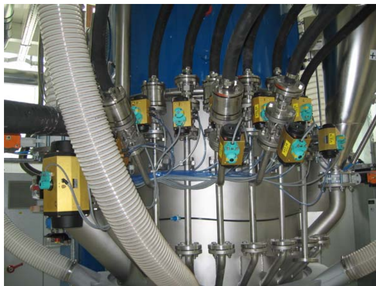
Liquid connections with check valves
